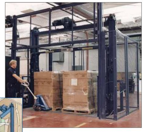
Pflow Series M Mechanical Vertical Lifts provide the added strength, speed and durability required for moving large, heavy loads. Series M Lifts are especially suited for multi-level applications and can be installed in new or existing buildings and unused elevator shafts. When it comes to vertical lifting, no challenge is too big, too heavy or too tall for Pflow. Vertical lifting is our business—our only business.
