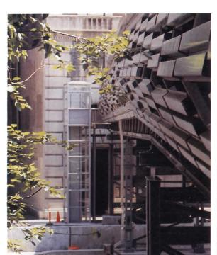
to 25 feet, we recommended a custom-designed vertical wheelchair lift with its own self-contained enclosure, ventilation system, landing doors, interlocks and cover dome. To my knowledge, a unit with these design parameters had never been built in North America. The biggest challenge was to design, manufacture and install these units in approximately 10 weeks. For this, I approached Savaria Industries, and they rose to the challenge.
