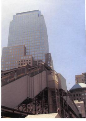
We took special care to make sure this steel structure is adequate, all loads including wind resistance were taken into account. The total height of the lift enclosure exceeded 34 feet. The drive mechanism was chain-hydraulic, and due to the amount of travel, a special auxiliary oil tank was designed to accommodate the hydraulic fluid.
